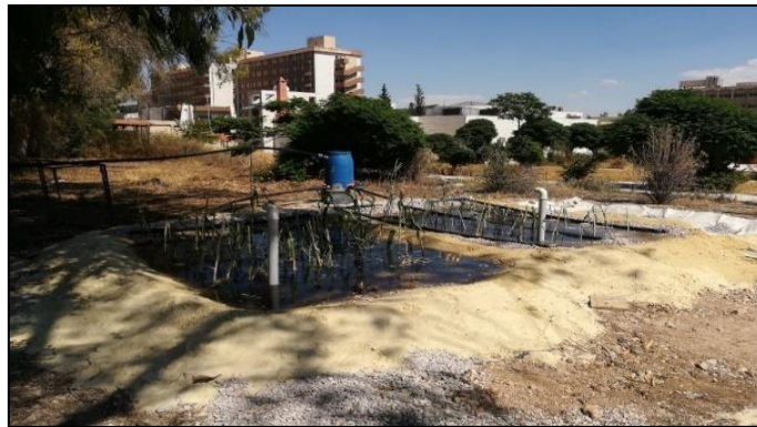
two treatment basins with artificial wetlands :)14( Figure (HSF,FSF).
