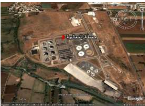
Figure (3) Aerial view of the sewage treatment plant in Homs city
