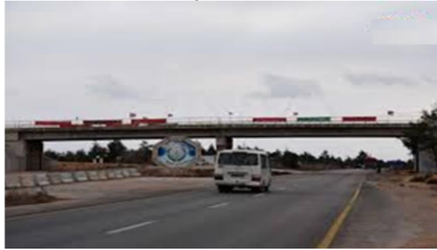
Fig (8). Al-Houla Bridge (a camera photo)
